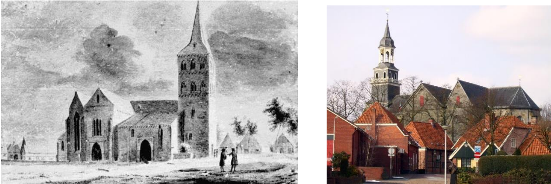
Fig. 3: The church in Ootmarsum. Left: the church around 1733 (a sketch attributed to Abraham de Haen); right: the church in March 2006 (Photograph: H.-U. Hillebrand, Gescher, click to enlarge).
